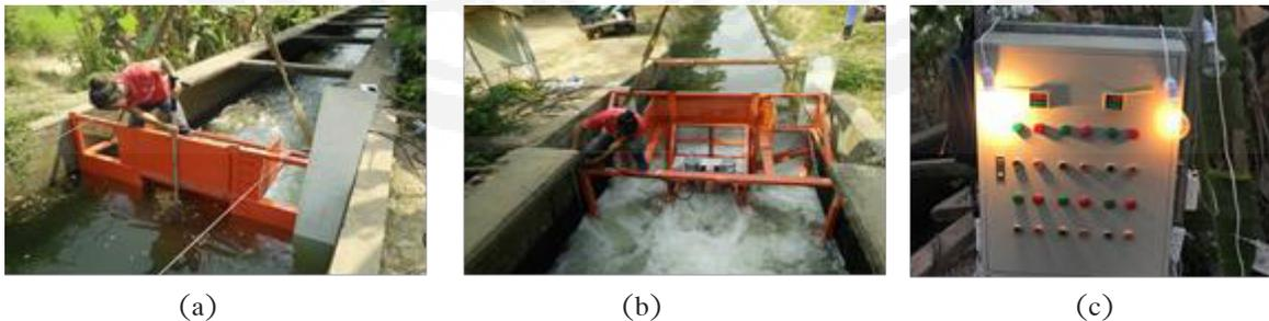
Figure 8 Installation and trial turbine system (a) measuring input water flowrate (b) measuring water head (c) display monitoring system
