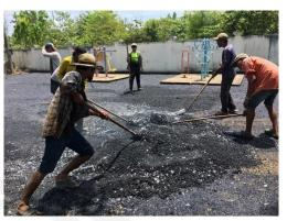
Figure 8 Mixing plastic bag waste with workers
