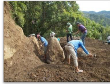
Figure 44 Men are removing a big stone. This difficult instance in a distant community where superior technology is absent will necessitate the help of others.
